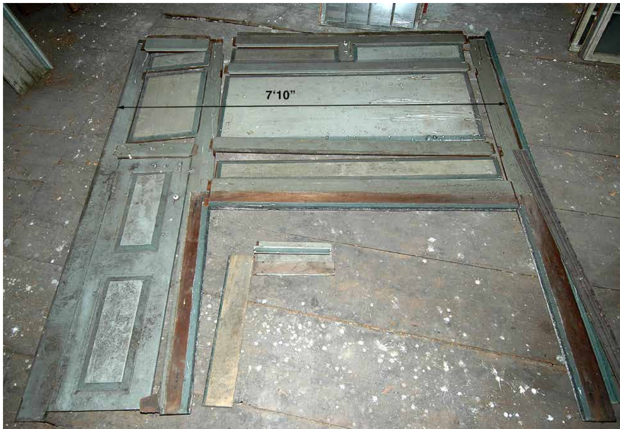
Photo 70: Mid-late 18th century paneling that is stored on the attic floor. There is no record of where it came from, but its 7' 10" width matches the original hall fireplace opening width suggesting it was removed from the hall in 1920. Its two tone color scheme is similar to the Victorian appearance of the hall chamber woodwork. That there are no marks from plaster lath on indicates it was still exposed at the start of the 1920 restoration. The bare wood around the fireplace opening suggests its molded surround had been removed to fit some later infill over the fireplace masonry.
