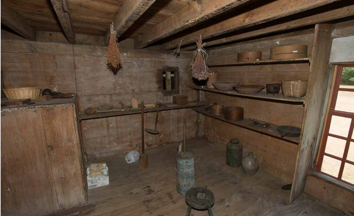
Photo 42: Photo of the north and west walls of the pantry in 2016. It probably had a plaster ceiling when originally constructed, as there is no remnant of whitewash above the bottom of the joists and on the wall girts.
